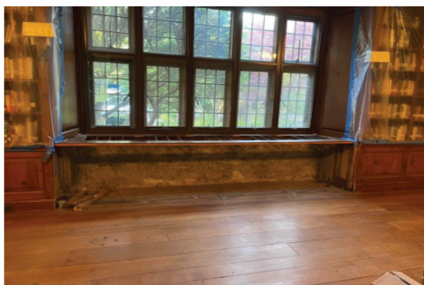
Removal of old radiators from Living Room
